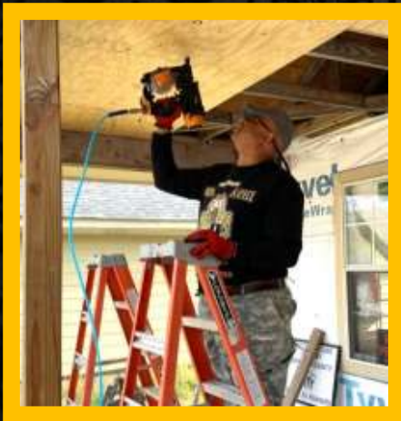
Bro. Kerry Taylor helping Habitat for Humanity with ceiling plywood
